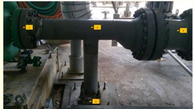
Figure 3 Some of measurement points on pump suction piping
