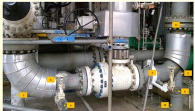
Figure 4 Some of measurement points on pump discharge piping
