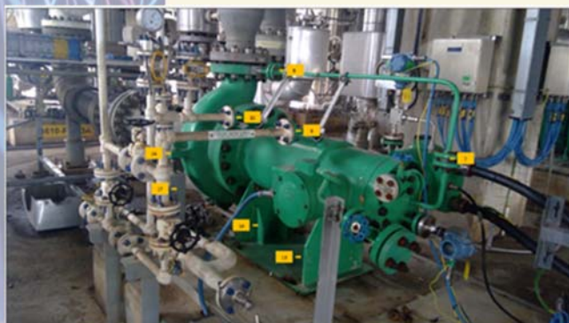
Figure 2 Some of measurement points on the pump body
