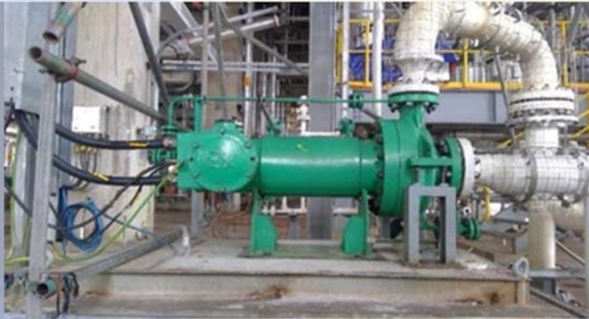
Figure 1 Pump package overview
