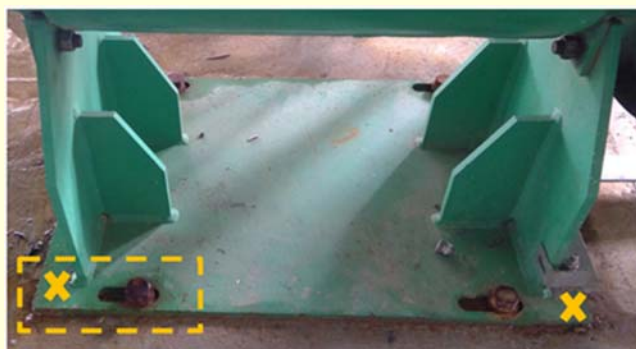
Figure 10 To add or re-positioning the hold down bolts
