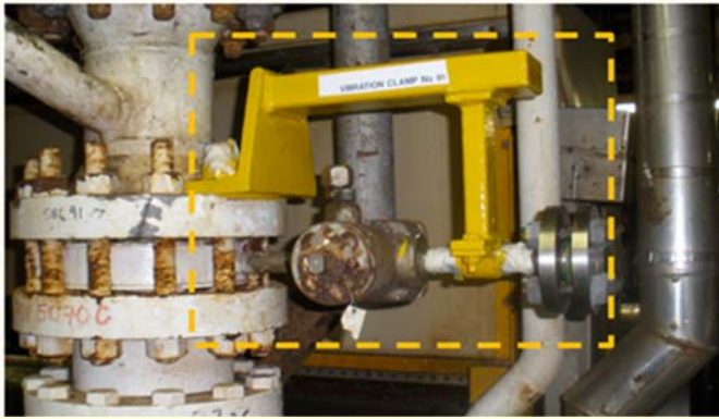
Figure 11 Additional support or braces for SBCs or flange
