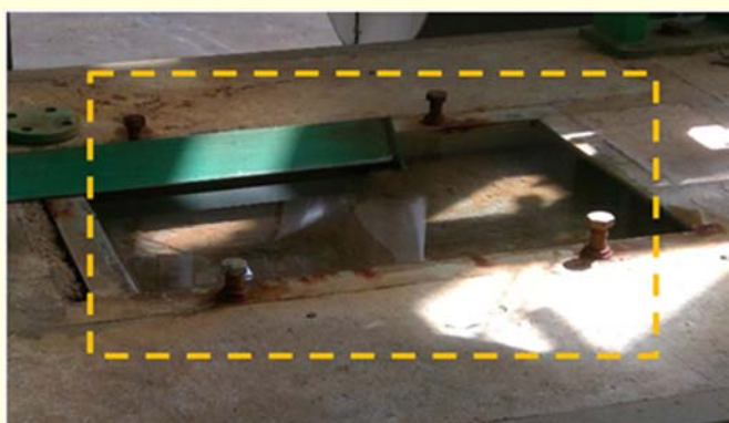
Figure 8 To grout the empty foundation under baseplate (at site)
