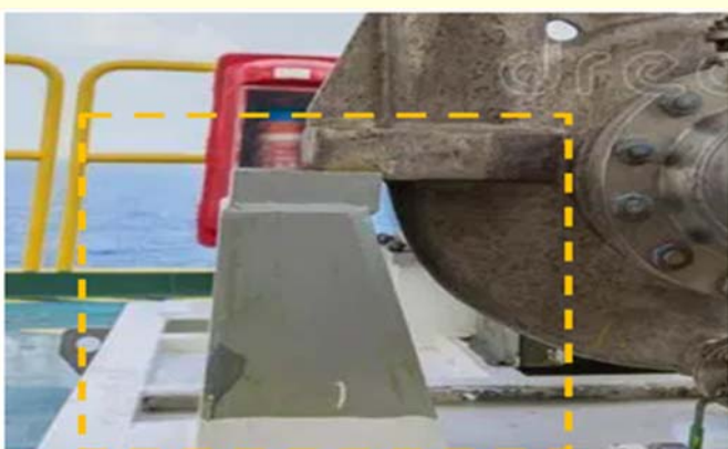
Figure 9 Example of pump support skid levelled with pump skid
