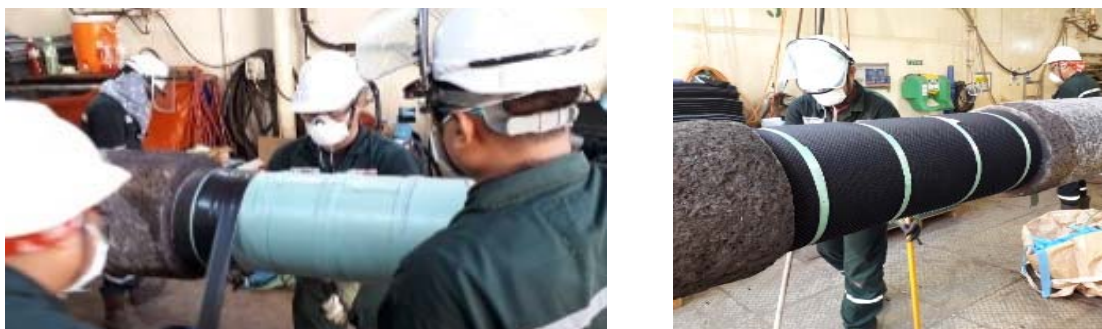
Figure 3: Innovative and Effective Field Joint Coating using Visco Elastic Self- Healing Product is a new technology that provides reliable and fast application during pipelay activity. It is a cold application without the need of hot source such as fire torch.
