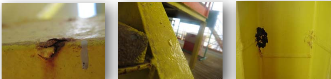
Figure 1: Some common coating failures seen offshore are blistering, paint sagging and hard to reach areas. It is important to continue to explore new coating technology such as thin-film technology to provide more advantages over conventional coating systems in term of surface tolerant, humidity level and etc.
