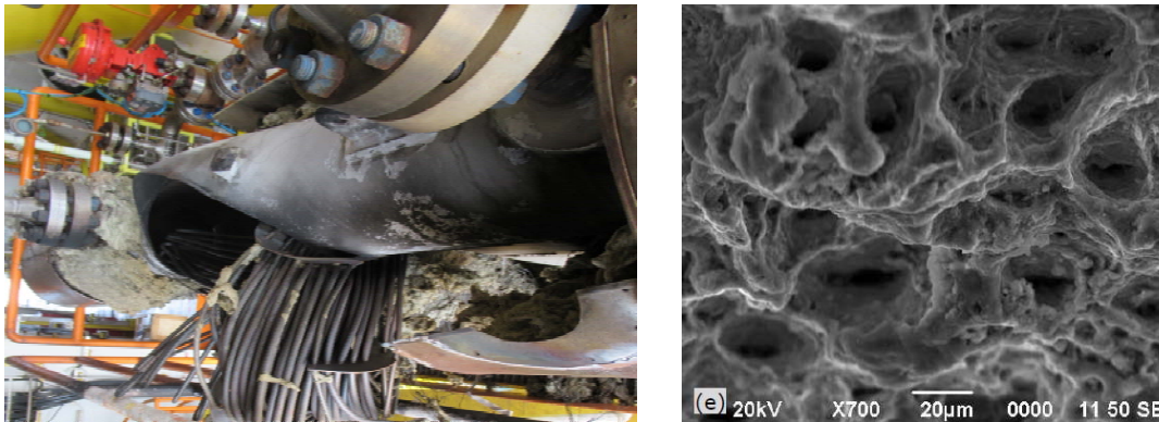
Figure 5: Level 2 Fitness for Service Assessment has been conducted together with the company, inspectors and 3rd party specialist. Metallurgical analysis of the ruptured gas preheater including visual inspection, fractographic, hardness, ferrite, SEM analysis, etc
