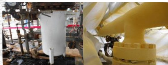
Figure 6: Pictures of Aerolon thermal insulative coating application on vessel and piping.
