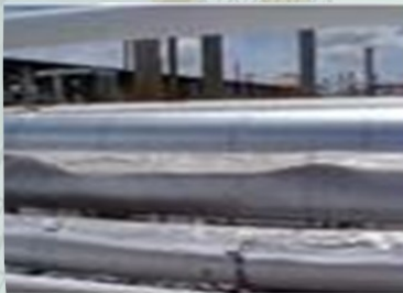
Figure 4: Personnel stepping on and damaging the cladding
