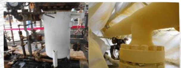
Figure 6: Pictures of Aerolon thermal insulative coating application on vessel and piping.
