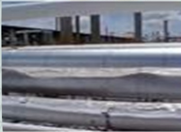
Figure 4: Personnel stepping on and damaging the cladding
